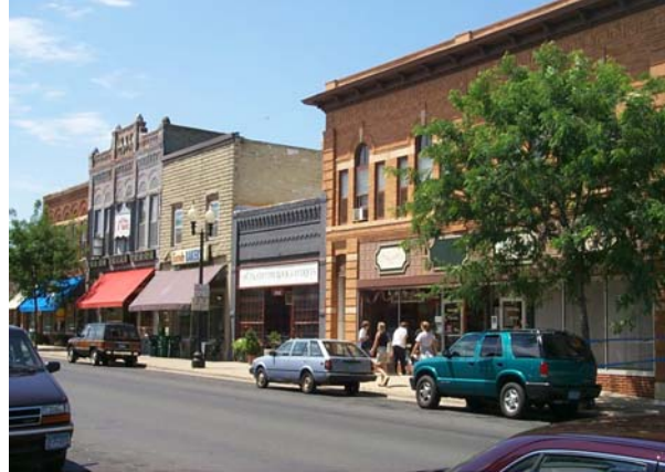
Example of a change in building facades and rooflines.
